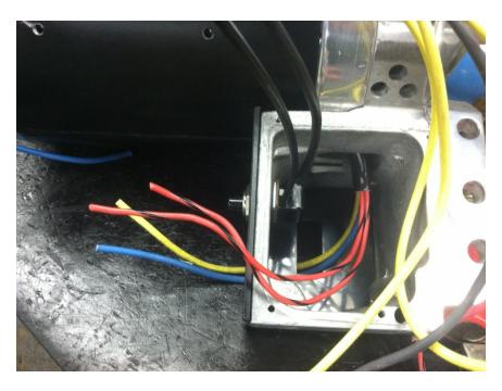
9. Remove the retaining nut from the momentary on switch (580C1-93) and install it into the back side of the front bearing housing as shown with the two wires coming out of the open side.
