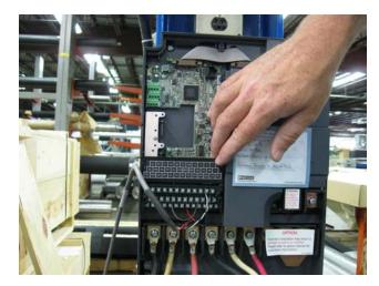
Replace the front cover of the VFD and tighten cover screws.
