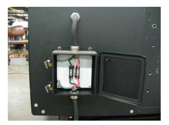
Ensure that wire colors match while installing on the terminal block.
