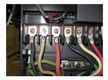
Attach the blower motor power cable using ring terminals to U, V and W terminals. Also attach the ground wire to ground terminal.
