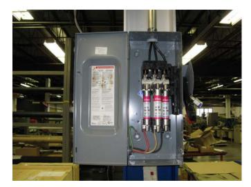
• Install incoming power cable using ring terminals as shown in the picture, the (3) incoming power wires are attached to L1, L2 & L3 terminals. Also attach the ground wire to ground terminal.
