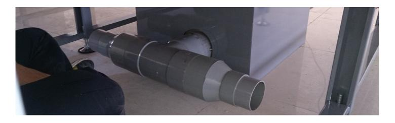
Connect flexible pipes to joints and lock up with metal ties
