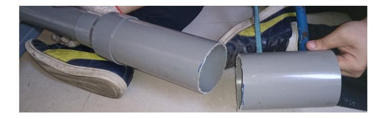
No glue needed for the lower head of L-shaped joint as connecting to the PVC pipe.
